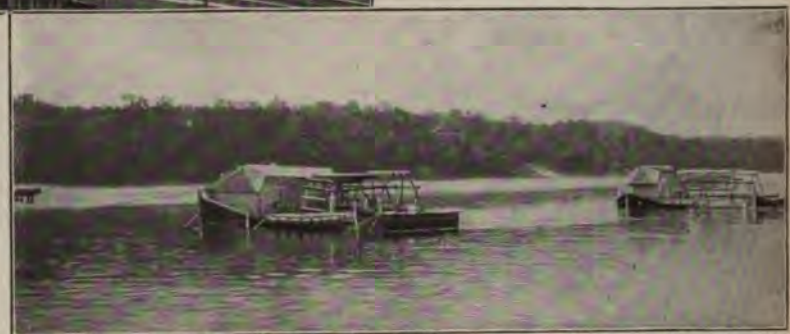
The Danube passing through the great plains of Hungary, above Budapest. The watermills which you see are built on boats anchored in the river. Between two boats is the great water wheel, which is turned by the force of the current and furnishes power to grind grain.
